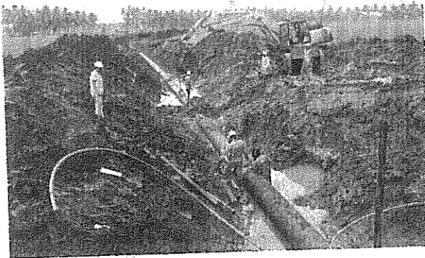
Gas pipeline being laid by GAIL near Bodasakurru in Amalpuram division in East Godavari. - PHOTO: B.V.S. BHASKAR
